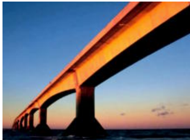
The Confederation Bridge spans the distance between Prince Edward Island and New Brunswick
